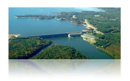
SCOPE OF WORK: This project is a \$46 million plus major renovation for replacement of turbines, restacking and rewinding of generators, replacement of GSU transformers and extensive balance of plant equipment. The general contractor is Andritz Hydro, Pointe Claire, Quebec, Canada. Koontz Electric Company was awarded a subcontract by General Electric for the balance of plant electrical work. The work consists of:
