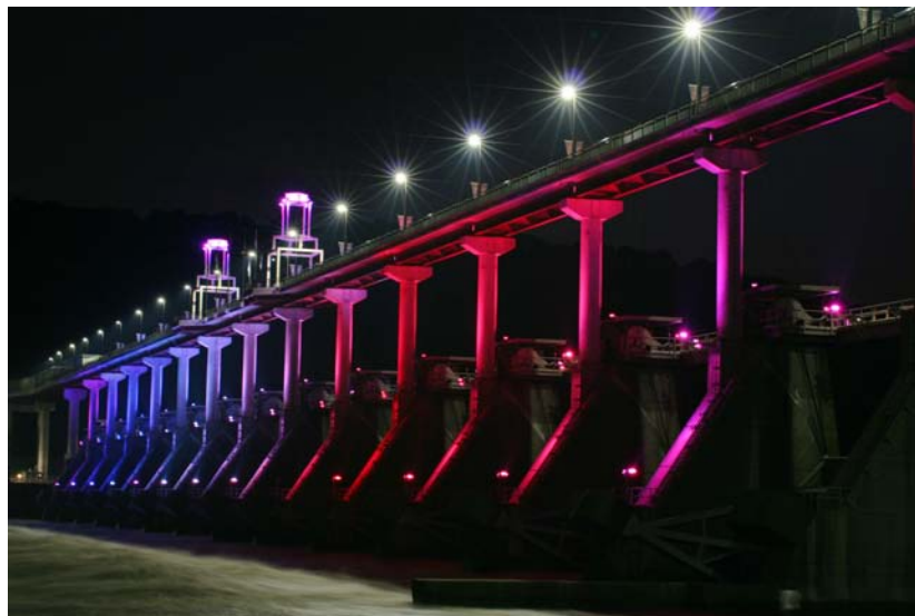
Koontz Electric Inc. of Morrilton says it is finding yet another niche in LED lighting, which it installed at the Big Dam Bridge pedestrian walkway atop the lock and dam at Cook's Landing spanning the Arkansas River.
